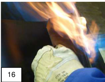
16 Warm one end of the adhesive side of the closure patch with a gas flame. Position the warmed side of the patch over the exposed edge of the sleeve.
