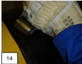
14 Roll on the overlapping area.
