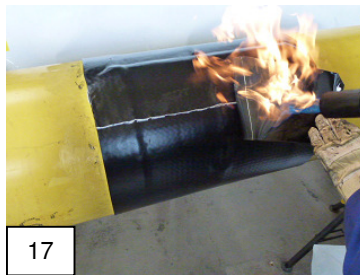
17 Continue warming up the adhesive side and position it over the whole sleeve width in the overlapping area.
