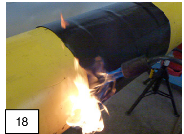
18 Continue warming up the adhesive side of the closure patch and position it over the whole sleeve width in the overlapping area.
