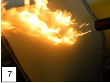
7 Remove approx. 300 mm of the release film from the whole width of the mitred end of the sleeve. Warm up the butyl rubber using the propane torch.
