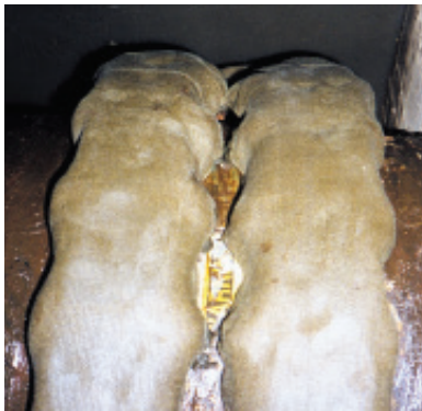
Densyl Mastic Blankets applied to flange pair.
