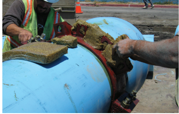
Coupling prepared with Denso MP Primer and Profiling Mastic prior to Petrolatum
