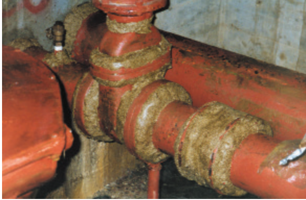
Denso Profiling Mastic on valve and coupling.
