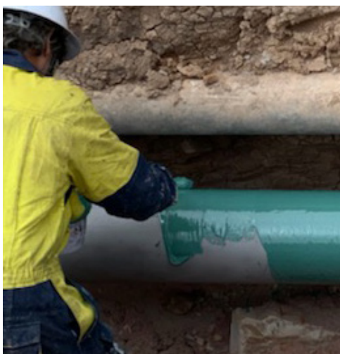
Denso Protal 7200 being applied to the pipe.
