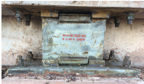
Bare roller showing no signs of corrosion
