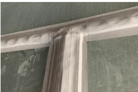
Denso FB30 Tape used to protect a water storage tank liner from construction bolts.
